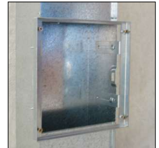
2 FLUSH MOUNTING SYSTEM (FMS) INSTALLED INTO BACK BOX
