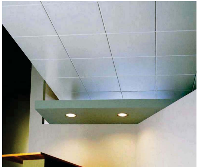
Acoustic Ceiling Installation
